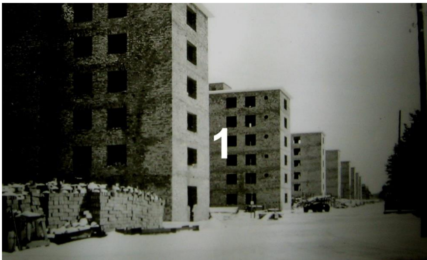
1. Building of the stairwell, winter 1938/39
